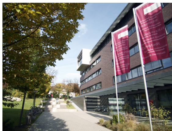
Building S3|20 seen from Rundeturmstraße
